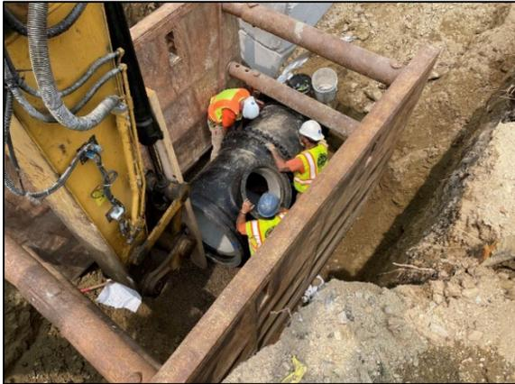
Installing the 36-inch by 20-inch Tee on Section 23 for Emergency Interconnection
