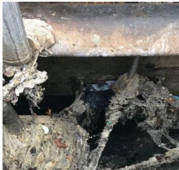
*Figure 4. Rag Buildup in Process Tanks*
