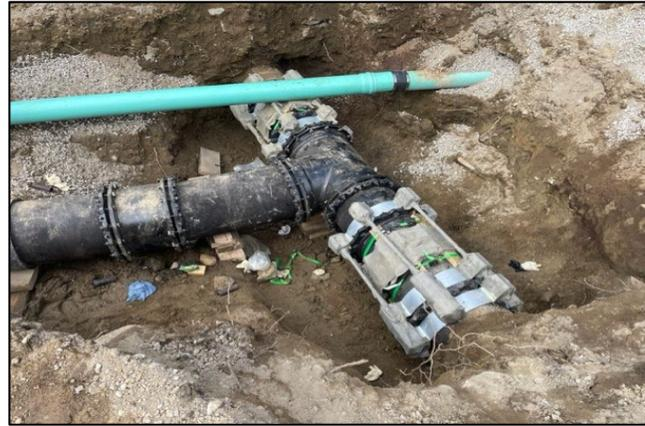
Completed Piping at the City of Newton's Existing 20-Inch Water Main
