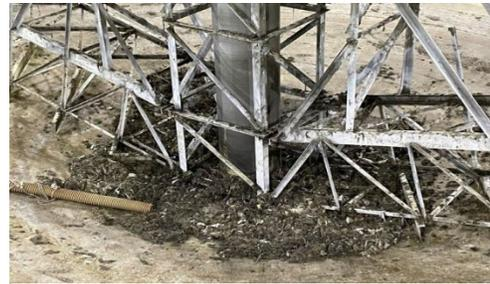
*Figure 3. Gravity Thickening Center Column Clog*
